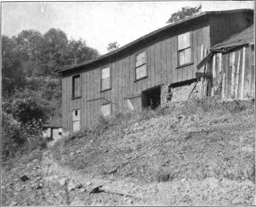
A. PUMPING STATION AT PARKER, PA.
